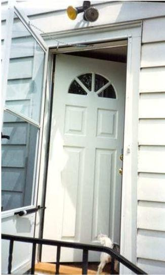
Exterior view of an arch type prime door and storm
